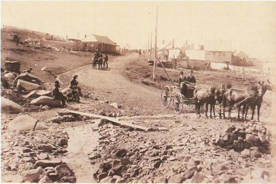
A country town begins. Many new towns scarred the landscape, especially in mining and forestry areas. The telegraph, to be carried on the poles in the centre of the picture, came early to new towns. Good roads were built later.
