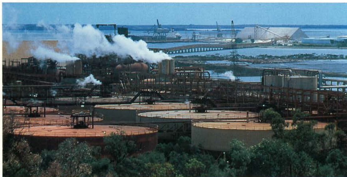
After extensions in 1973 the alumina refinery at Gladstone was the largest in the world. The refinery dominates Gladstone's townscape. Photograph by John Houldsworth, 1981.
