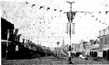
MOORABOOL STREET, GEELONG.
